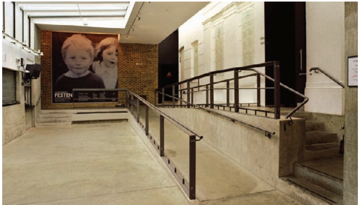
Access improvements at the Almeida Theatre, London, were part of a larger project. The foyer ramp gives access to the stalls seating area.
