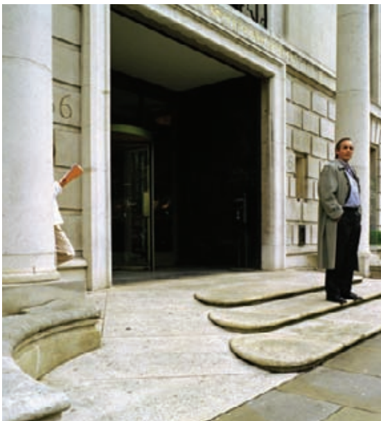
This elegant solution at the Royal Institute of British Architects overcomes a small change of level at the entrance.
