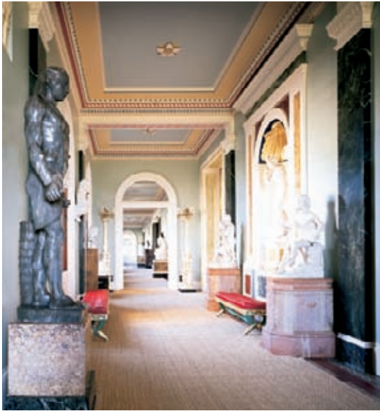
A Minton tile floor, such as this one underneath matting at Osborne House, is particularly vulnerable to both foot traffic and wheelchairs and needs to be protected.
