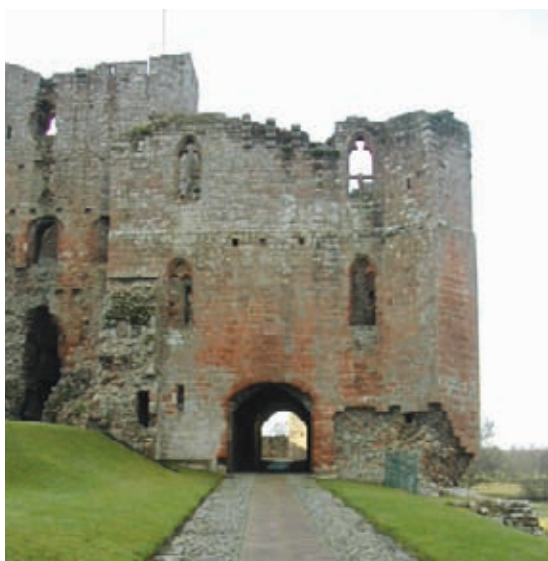
Cobbles and setts can be difficult for ambulant disabled people to walk on, especially if they are rough, uneven or open-jointed. At Brougham Castle, Cumbria, a smooth path is laid across an uneven surface to create a more accessible route.
