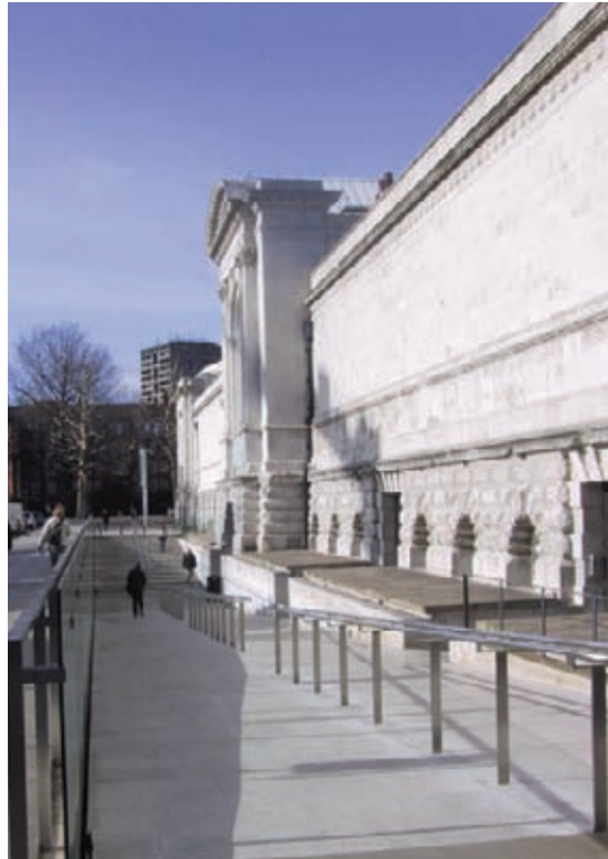
A new accessible entrance at Tate Britain has wide steps and ramps.
