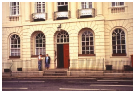
At Ripon Town Hall the whole pavement has been ramped up to threshold level over the original steps, part of a scheme that included the addition of a lift and accessible toilets inside. Railings have been added because of the increase in kerb height, but no handrail has been provided for the steps.
